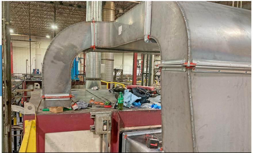
The ductwork coming off the top of the fan was directed straight down and tied into the ductwork on the inside of the paint booth.
